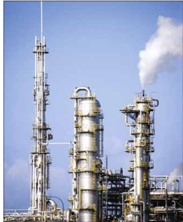
Columns of a refinery
