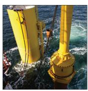
This segmental bushing, made of ZX-750V5T (Ø700 mm), guides and leads into water the floating weight of 28t in a deep-sea hammer. This extreme stress subjected part operates in unlubricated conditions, with a 50 Hz impact frequency and a drop height of 1 m.
